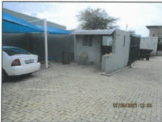
General external view of the gatehouse
