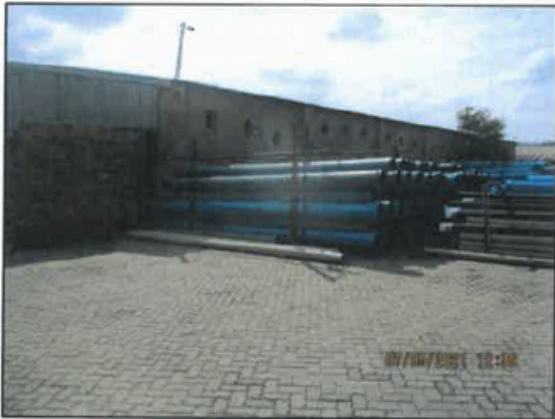
General view of the secure on-site open storage (Note the 80mm interlocking concrete brick paving)
