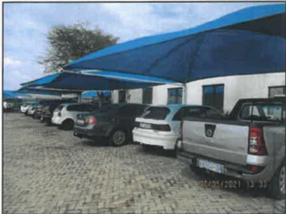
General external view of the shade cloth carports and the administration offices in the background
