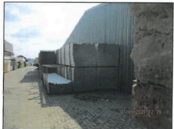
General view of the secure on-site open storage (Note the 80mm interlocking concrete brick paving)
