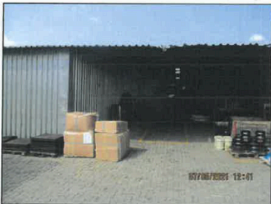
General external view warehouse and the attached covered lean-to
