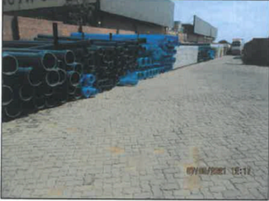
General view of the secure on-site open storage (Note the 80mm interlocking concrete brick paving)
