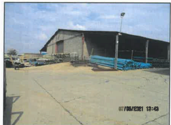
General external view of the warehouse and the attached lean-to
