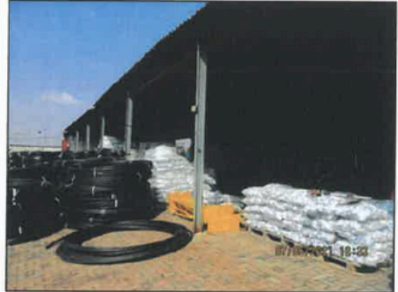
General view of the attached covered lean-to for the warehouse
